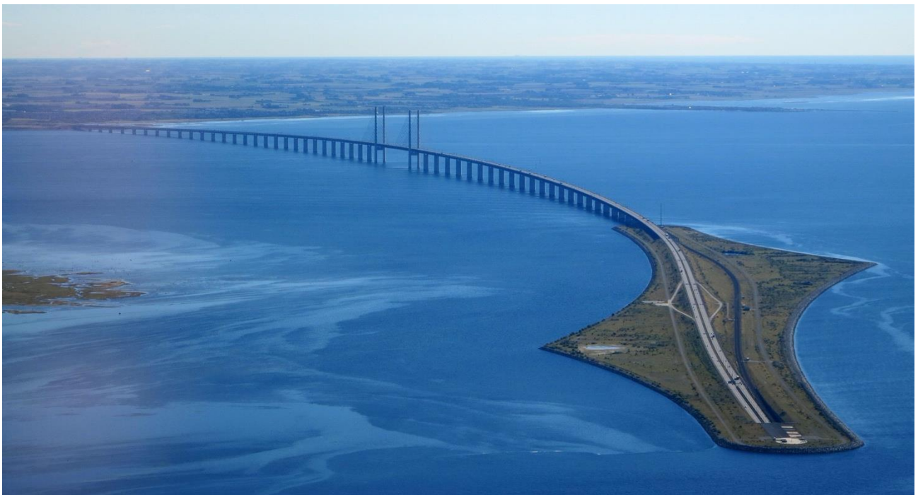
The man-made island of Peberholm: forms the system transition between the Øresund Bridge and the Øresund Tunnel and is located in the center of the 16 km long road and rail link between Copenhagen and Malmö.
